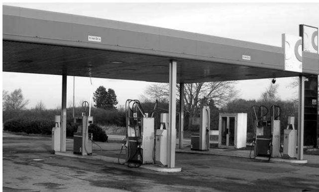
Figure 2: Photo of one of the measurement sites. OKQ8 gas station in Södra Sandby, Sweden.
