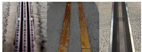
Fig. 2. Illustration of different road-bound conductive ERS solutions.
