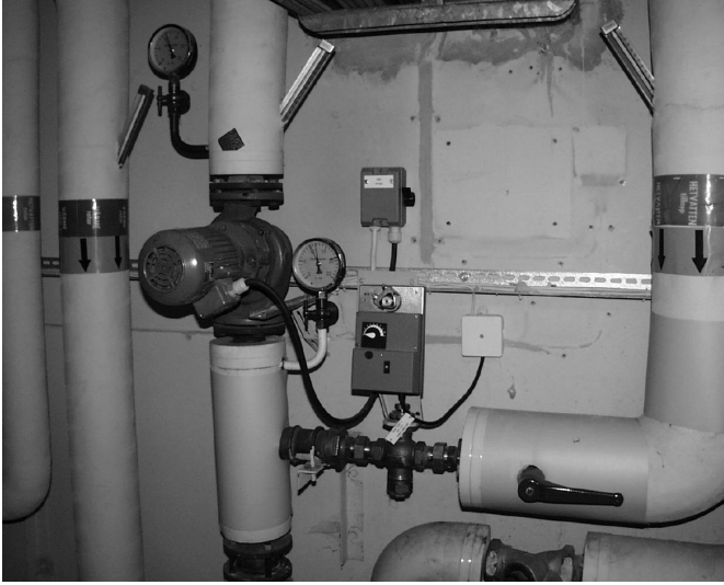
Figure 5. The control valve for the heating/ventilation system.
