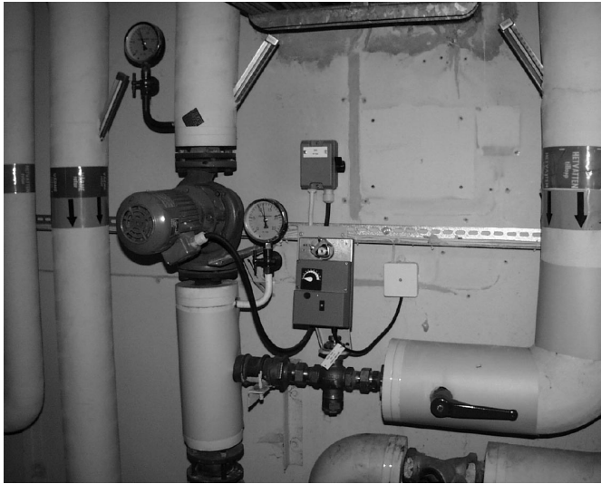
Figure 5. The control valve for the heating/ventilation system.
