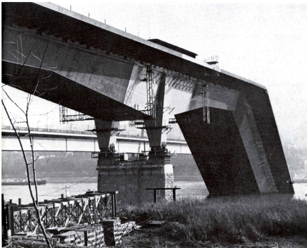
Fig. 8. Collapse of steel box girder during cantilever construction, Rheinbrücke, Koblenz, 1971, Source: Ref. [31].
