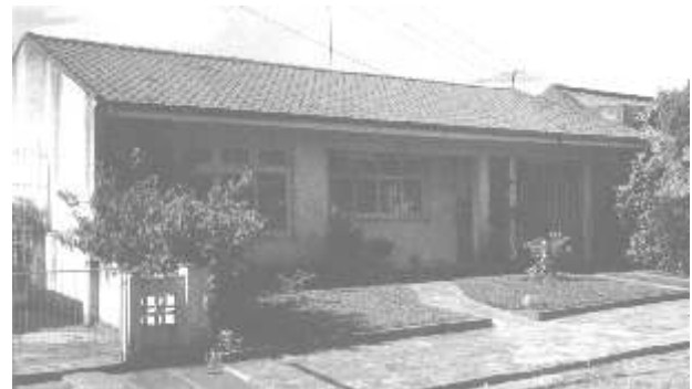
Fig. 37 Above: House in Porto Alegre, Brazil, built with the “Climatex system” (Fig. 36) with prefabricated wall elements of woodwool slabs and concrete.
