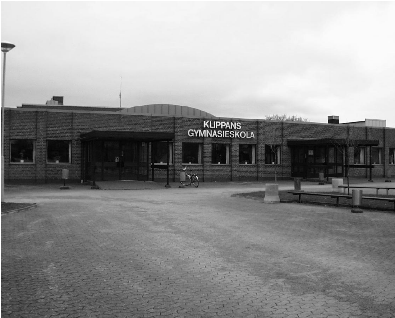
Figure 5.8 The school in Klippan.
