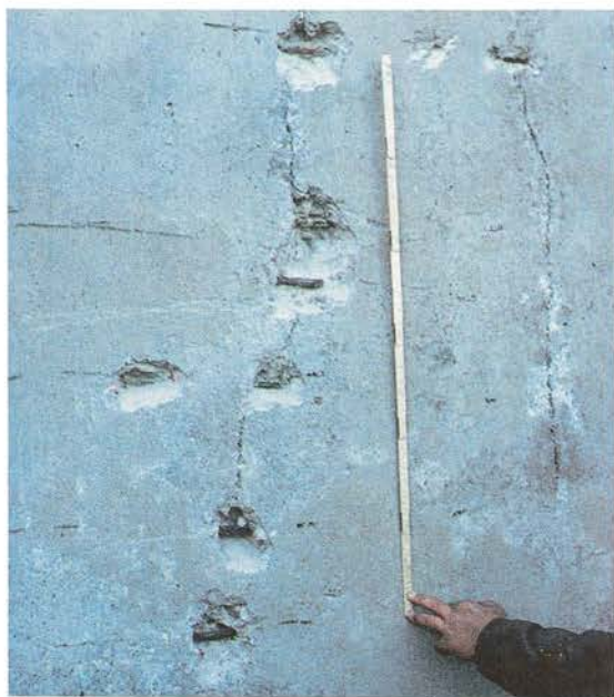
Photo 5. Photo of silo. Concrete chipped away to expose reinforcement in crack. Average centre-to-centre spacing 250 mm. Stipulated spacing 120 mm.
