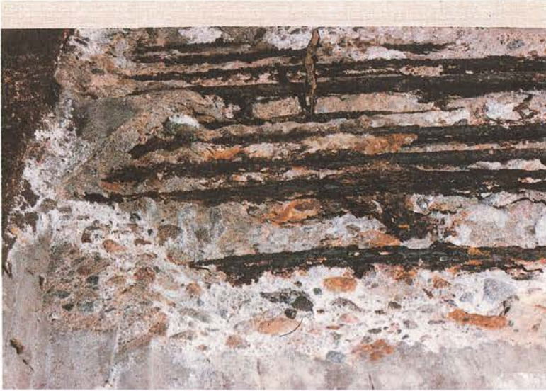
Photo 39. Corrosion of reinforcement in a traffic facility called Slussen in Stockholm where chlorides from road salt had initiated the corrosion process.
