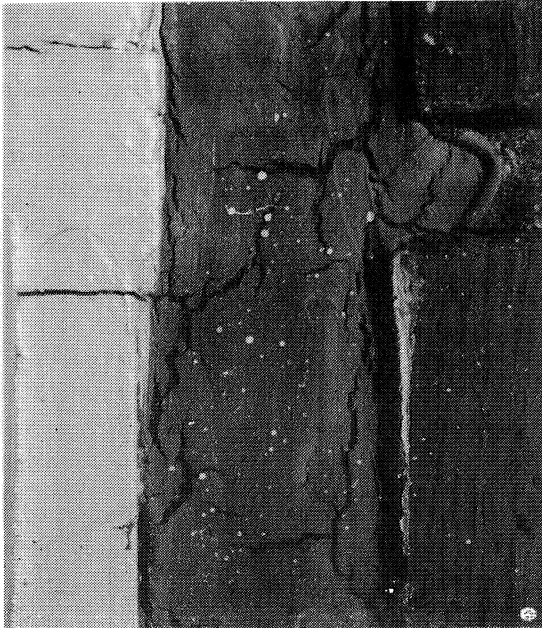
FIG. 6.2 Deep cracks in a 12 year old polysulfide-based sealant (50 0 Shore A). The joint is located indoors at a constant temperature of about +22 °C.
