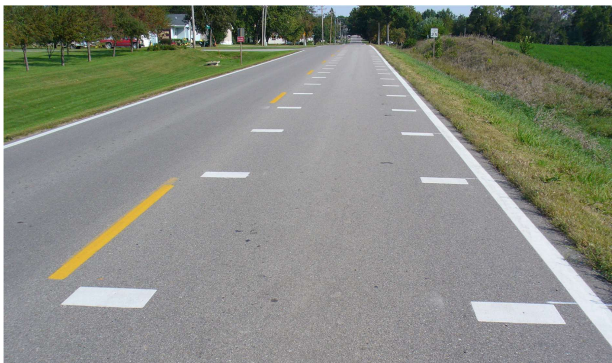
Figure 16. Transverse pavement marking bars (Fitzsimmons et al., 2009).
