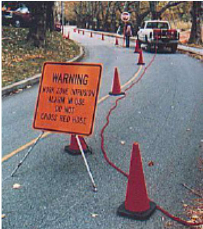
Figure 28. Pneumatic tube incursion alarm (Wang et al., 2013).
