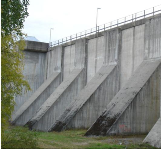
Figure 2-2 - Buttress dam at Stornorrfors.
