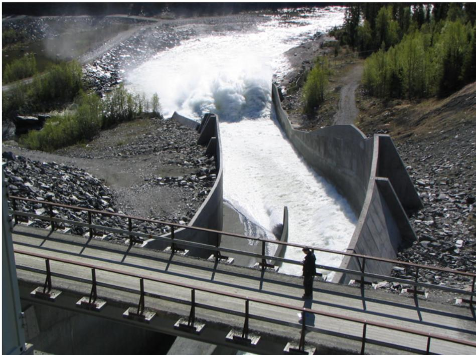
*Figure 6-1 - Ajaure spillway chute during discharge test.*
