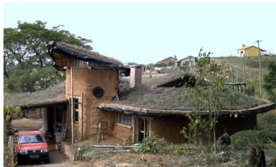
Figure 3.3: Complex self-constructed green roof (Krebs, 2005)
