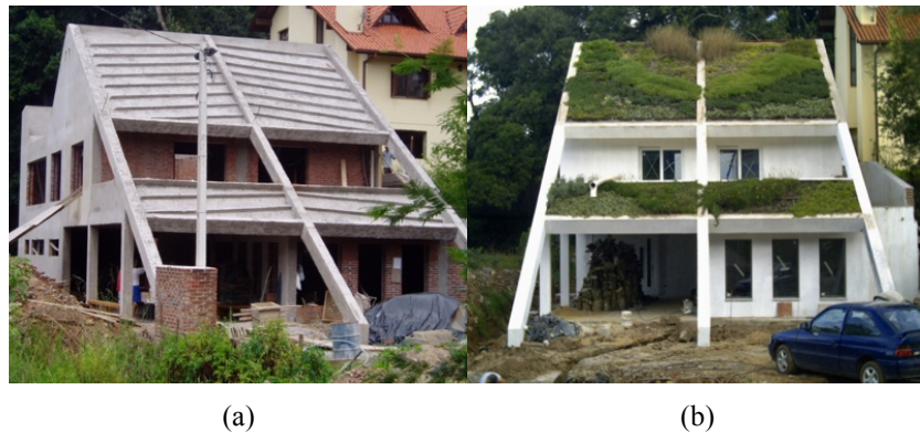
Figures 3.16 (a) and (b): Roof slab with barriers integrated, in a green roof in Nova Petrópolis, Brazil (The author, 2005)
