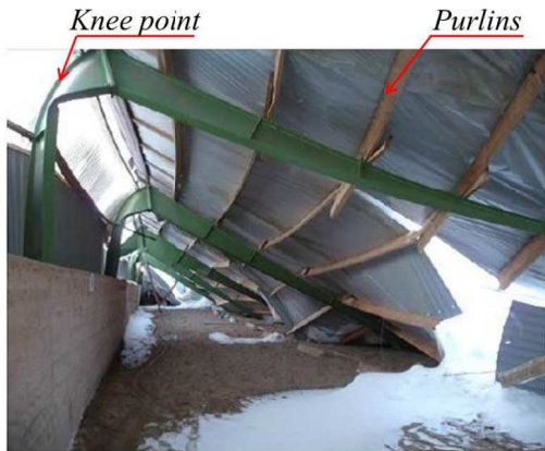
(a) Collapse that occurred during the winter of 2010/11 in Sweden (Johansson et al. , 2011). The frames were stabilized laterally by the use of purlins made of wood.
