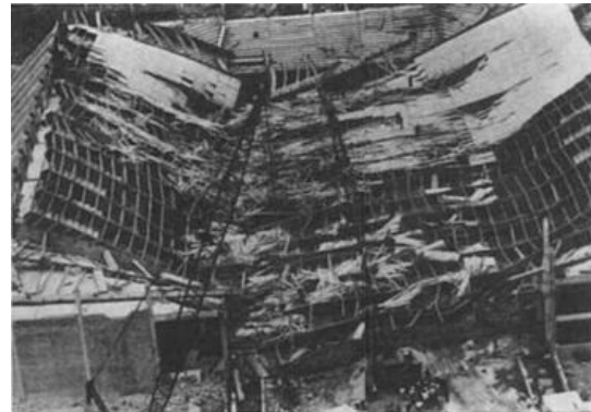
(b) A picture taken after the collapse. Note that there is no visible braced bay.
