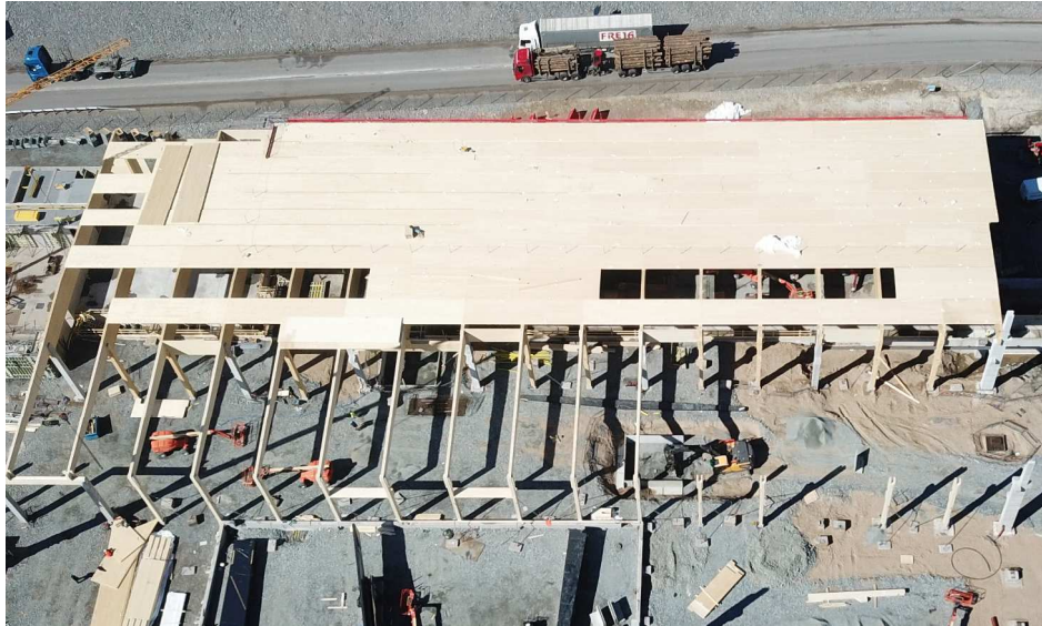
(a) The structure as seen from above.
