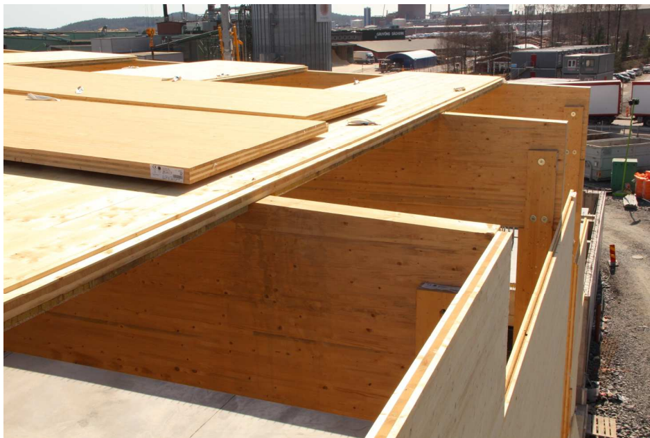
(b) A close-up picture of the CLT-decking.
