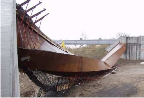
(a) A picture of the collapsed bridge.
