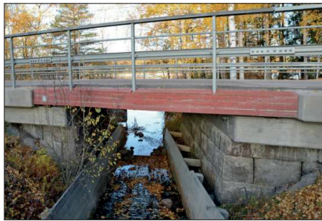
Figure 2.2: Damaged cross-laminated timber bridge. Photograph courtesy of A. Pousette & P.A. Fjellström.
