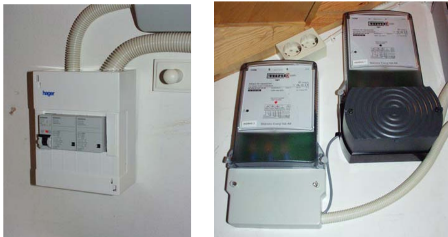
Figure 4.15. Control relay and extra meter
