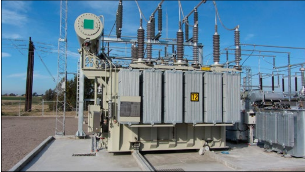
Figure 2. Picture of a conventional and typical 130/20 kV 40 MVA power transformer unit. A 63 MVA unit is physically slightly larger. [Ulf Lager E.ON Elnät Sverige AB]
