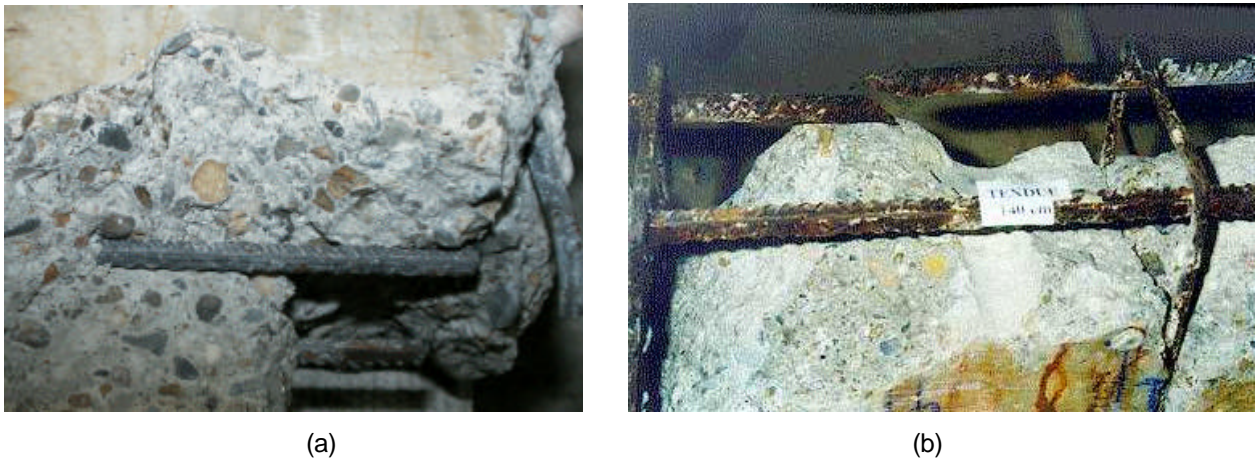
Figure 5: Comparison of the state of corrosion between two reinforcements of two 12 year-old reinforced concrete beams. For both beams, the chloride rate at the vicinity of re-bars is the same and is higher than the chloride threshold currently accepted [10]. In the photograph on the left, absence of corrosion can be assigned to the good quality of the steel-concrete bond, whereas in the photograph on the right, corrosion of the reinforcements is related to preliminary mechanical damage to the steel-concrete bond [9].
