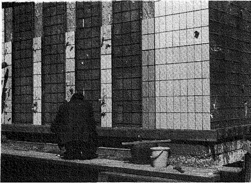
Figure 1.3.2v. House II, south wall: tile fixing on the column elements
