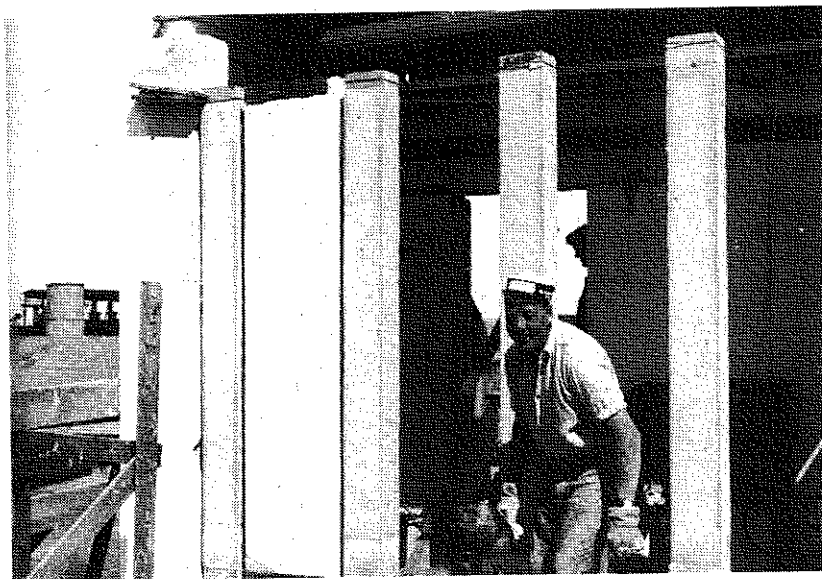
Figure 1.3.2t. House II, south wall: removing the forms from the concrete columns and raising the aerated concrete elements
