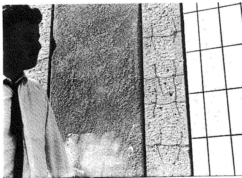
Figure 1.3.2u. House II, south wall: a splashed aerated concrete wall element and a splashed concrete column element with its anchoring wires
