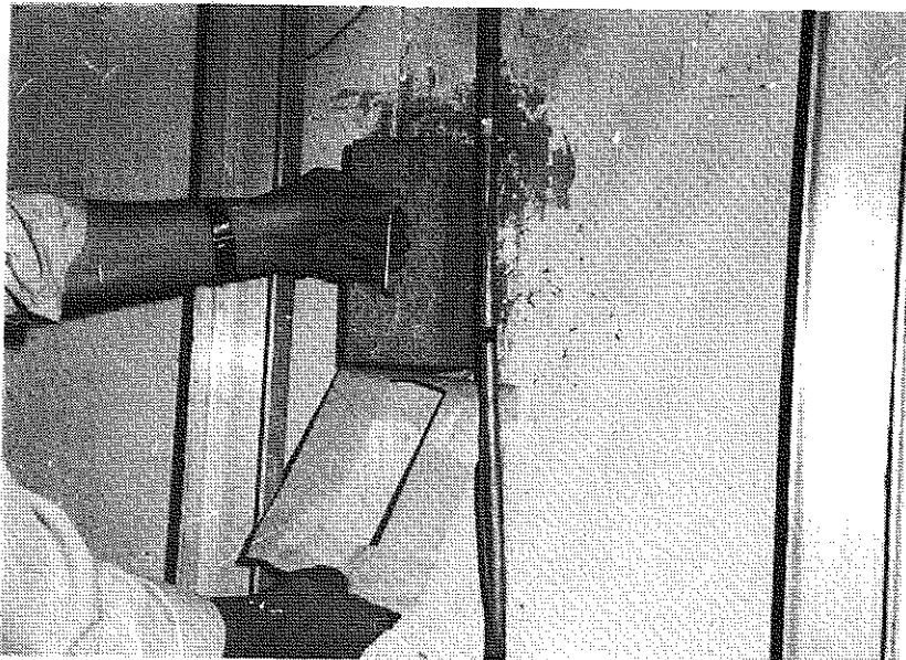
Figure 1.4.4e. The concrete test wedge in wall element no. 25, House I
