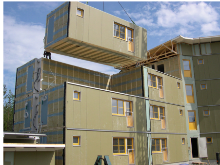
Figure 3. Modular house production.
