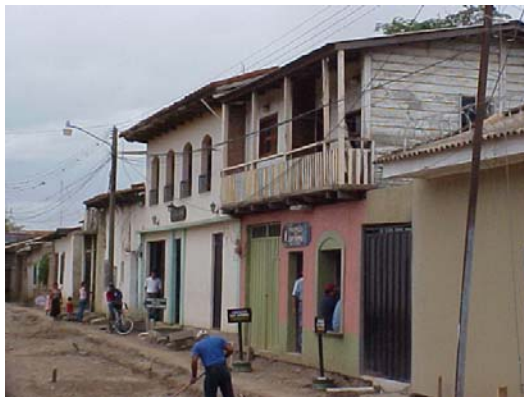
Partial view of the existing structures
