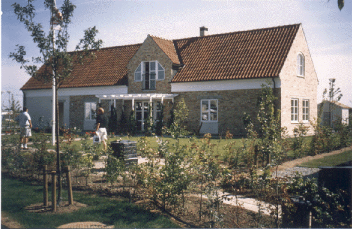
Figure 1. The Recycled House, build 1997 (Architect P.Lewis Jonsson.)
