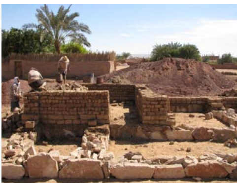
Figure 5.23 Wall construction phase.
