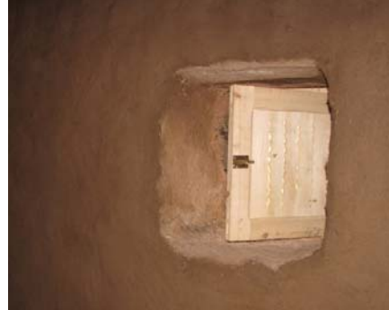
Figure 5.37 The window designed by Balat inhabitants and made by a local carpenter.
