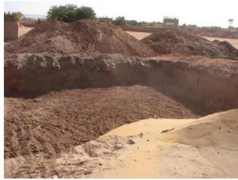
Figure 5.16 The site after digging.
