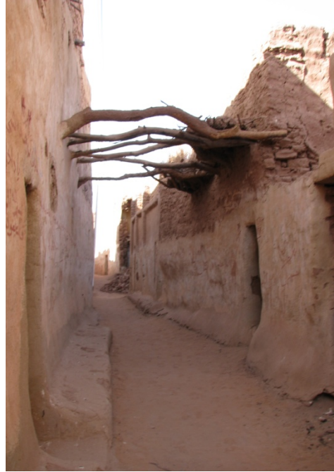
Figure 4.14 Example of shaded facades in narrow alleys.
