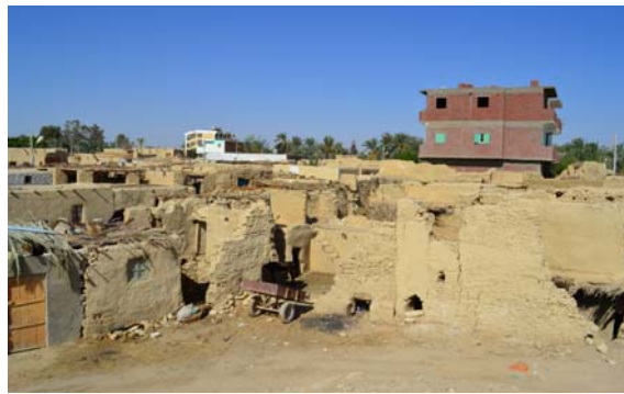
Figure 1.1 Deterioration of vernacular architecture and replacement of Karshif (salt rocks and clay) vernacular houses with concrete skeleton and fired brick ones in the Siwa oasis.
