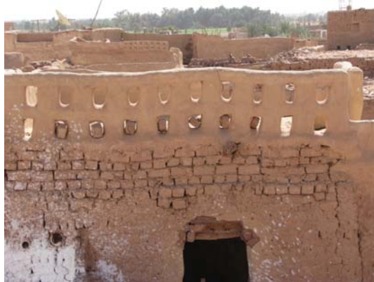
Figure 4.50 Example of exterior fences (parapets) in the roof floor made from mud brick .
