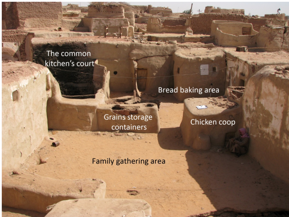
Figure 2.33 A floor constructed on a roof in order to extend a house, with four families sharing facilities such as a common kitchen, chicken coop and wheat storage, Dakhla oasis.
