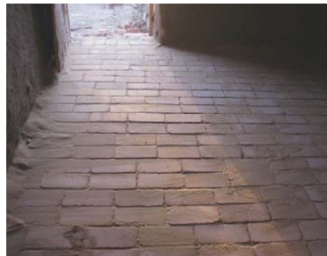
Figure 5.35 Sand floor tiles after finishing.
