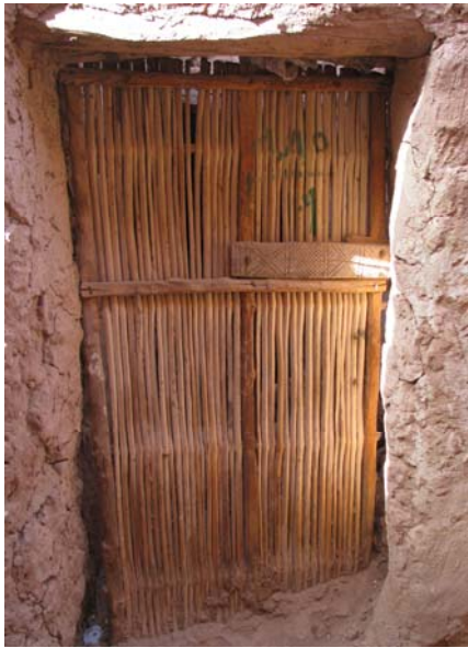
Figure 2.34 Doors in the Dakhla oasis made from palm tree ribs or reeds and the wooden key and lock are made from building construction wood leftovers.
