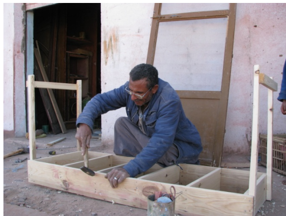
Figure 5.11 Kamel, the local carpenter in Balat, while working on implementing the new mould of size 50cm x 25cm x 15cm .
