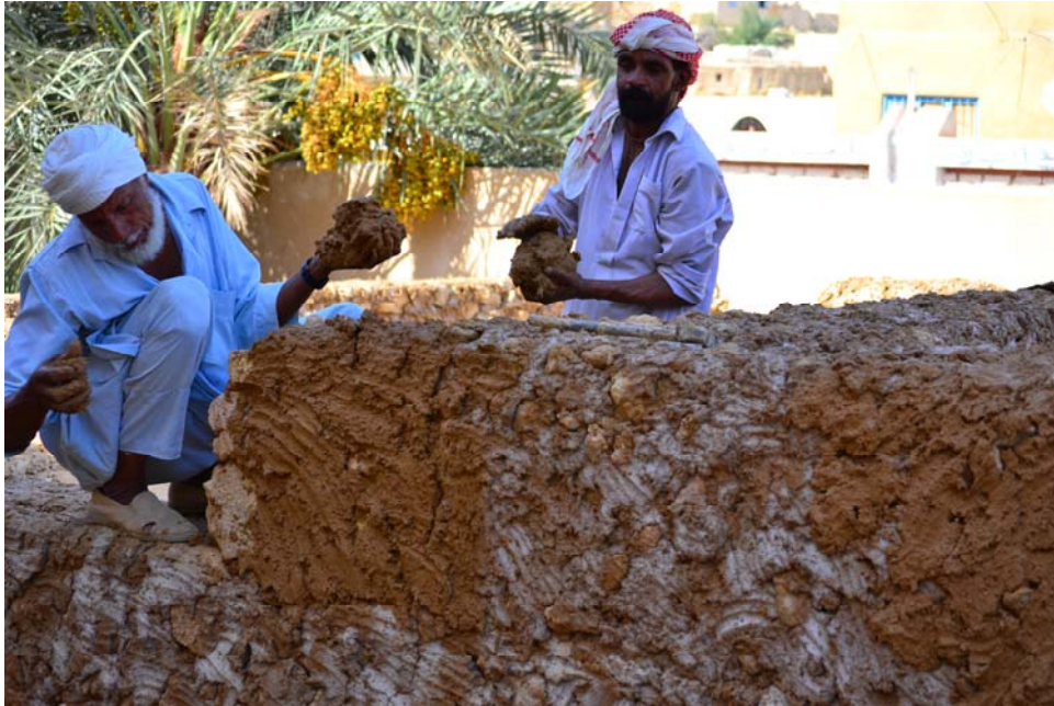
Figure 2.15 Vernacular builders in the Siwa oasis using salt blocks (Karshif) and mud. Roof construction is palm wood and mud brick.
