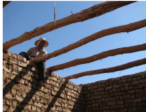
Figure 5.26 Placing the wood logs on the walls.
