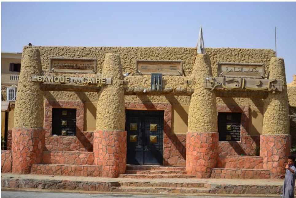
Figure 2.16 Local bank branch designed and constructed by The Siwa Sustainable Development Initiative with earth vernacular building technology in the Siwa oasis using Karshif. According to the designer, the building passed safety and security bank tests in 2008.
