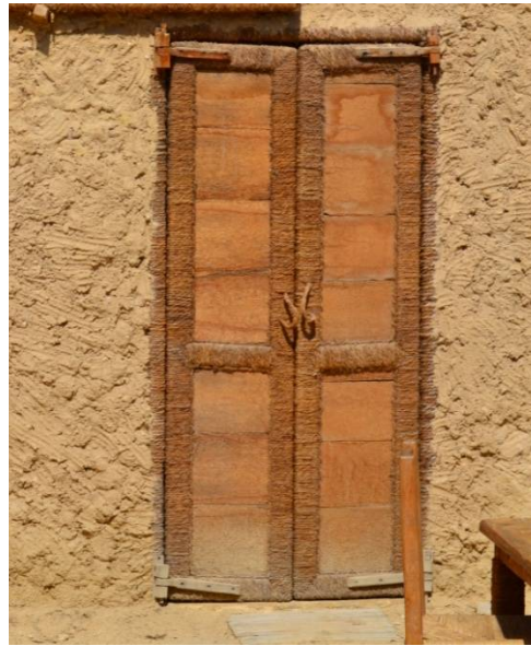
Figure 2.35 Doors in the Siwa oasis made from building construction palm wood leftovers and the door frame and door lock are made from ropes made from palm tree raffia fibers.
