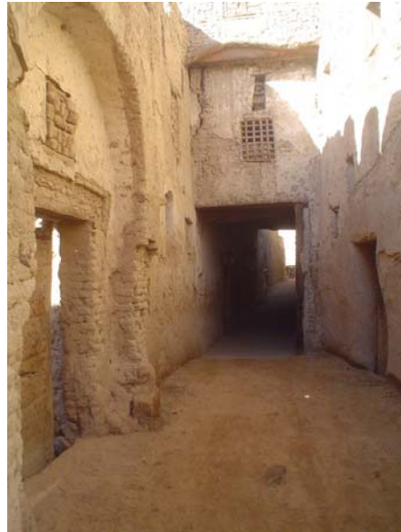
Figure 2.28 Shaded building facades in the Dakhla oasis.
