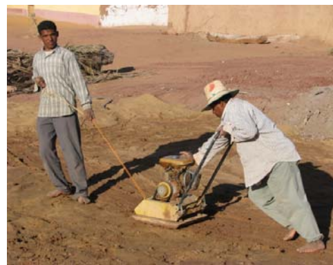
Figure 5.18 The site during soil replacement and compaction.
