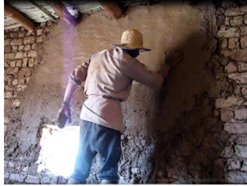
Figure 5.31 Plastering layer is smoothen by wet hand.
