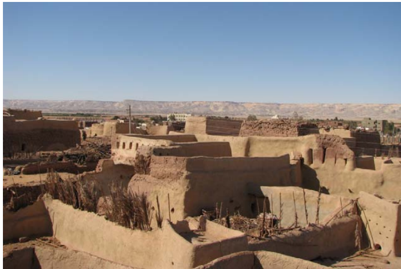
Figure 4.20 Composition of masses and typological architectural formation of dwellings in Balat. Inhabitants adjusted local materials to the purpose of connecting houses in delicate relations among houses' roofs.
