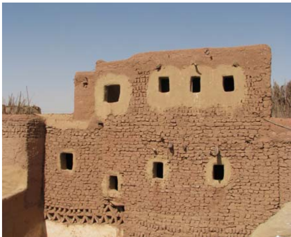
Figure 4.15 Different windows / openings in Balat houses.
