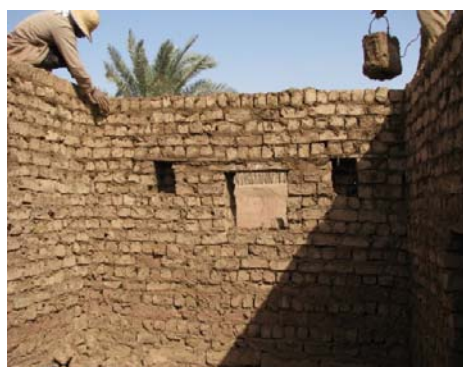
Figure 5.24 Windows and niches during wall construction.
