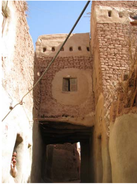
Figure 5.3 Shaded alley and a room bridging a street (Sabat) in Balat in the Dakhla oasis.
