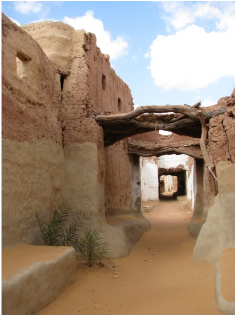
Figure 4.23 Built-in mud brick benches (Mastaba) is a main feature in the streets in Balat. They add an aesthetic touch to the townscape.
