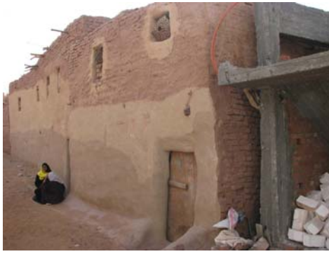
Figure 1.3 Replacement of mud brick vernacular houses with concrete skeleton ones in the Dakhla oasis.
