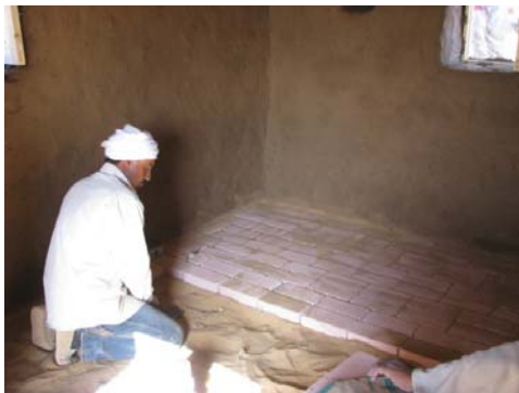
Figure 5.34 Floor making using sand tiles.
