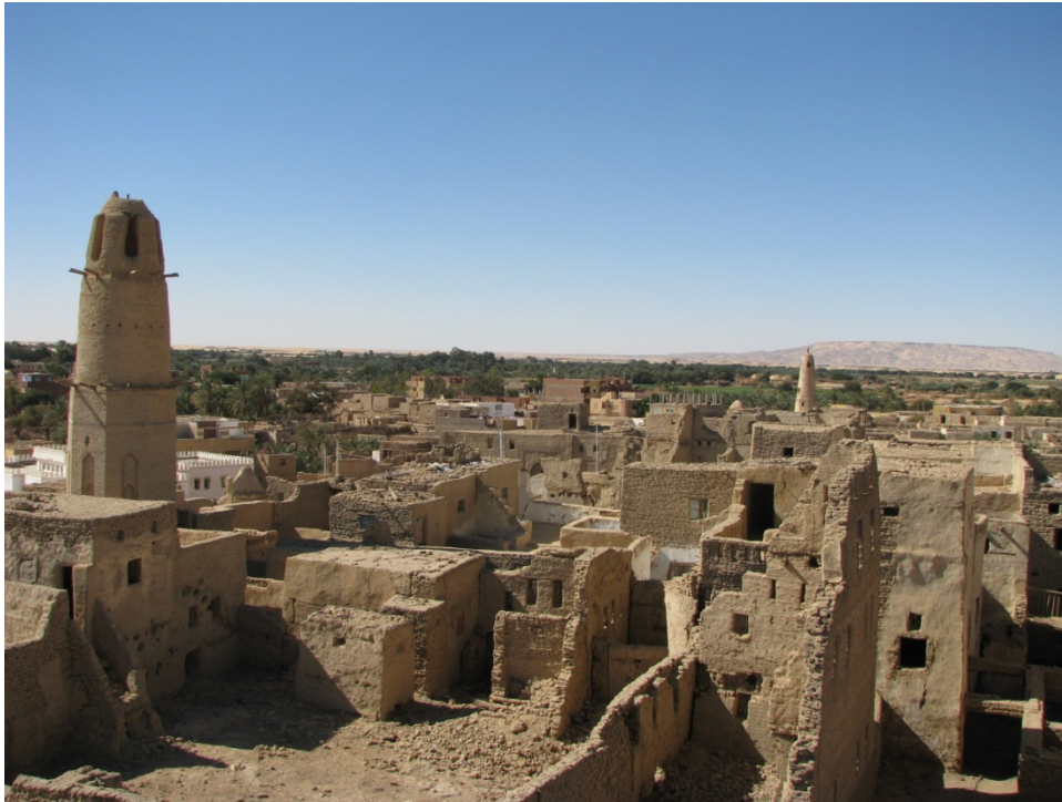
Figure 2.31 Example of a compact structure of a desert vernacular settlement with farm lands and cemeteries lie on the outskirts of Al Qasr town in the Dakhla oasis.
