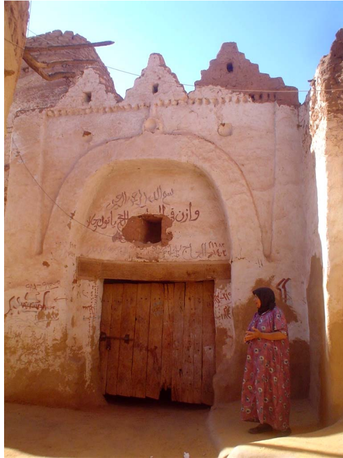
Figure 4.29 A house facade in Balat shows the human scale and aesthetic proportions.
