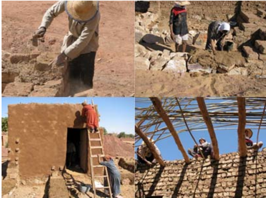
Figure 5.39 The built room of the neo-desert vernacular model house during different work phases.
