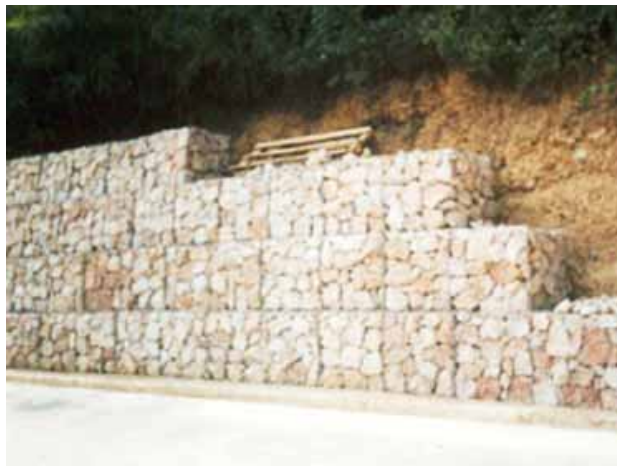
Slika 10. Gabionski zid (Soldo, 2010)
