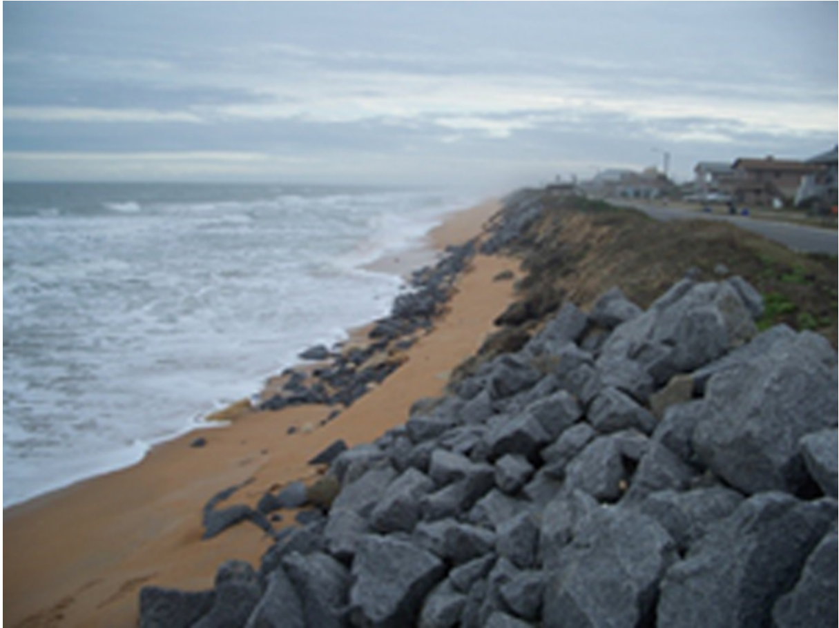
Fig. 3. The intersection of coastal erosion, loss of fore-dune vegetation, infrastructure placement and erosion prevention measures (failing rock revetment). Author's photo: January 2014. Taken from dune over-walk, looking south at South 18th Street in Flagler
