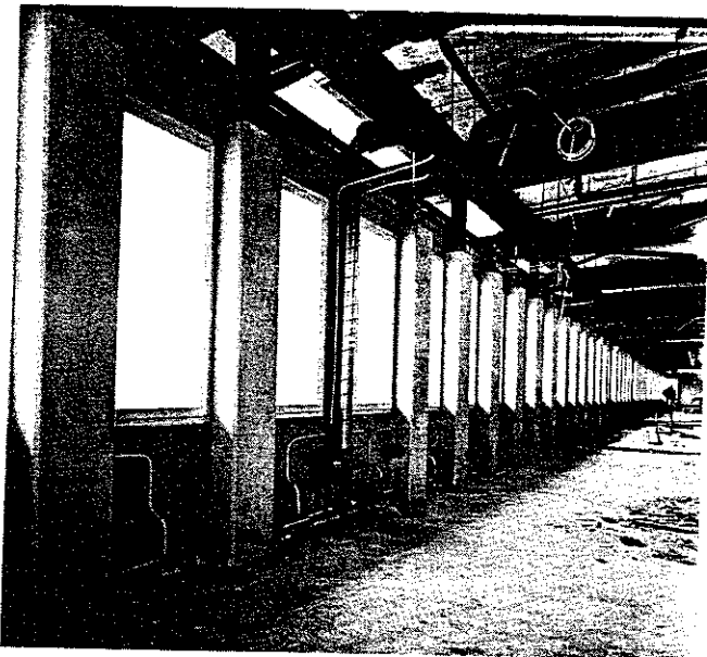
Fig. 11.1.8 a. Facade columns with fire insulation in the form of prefabricated gypsum plaster sections
