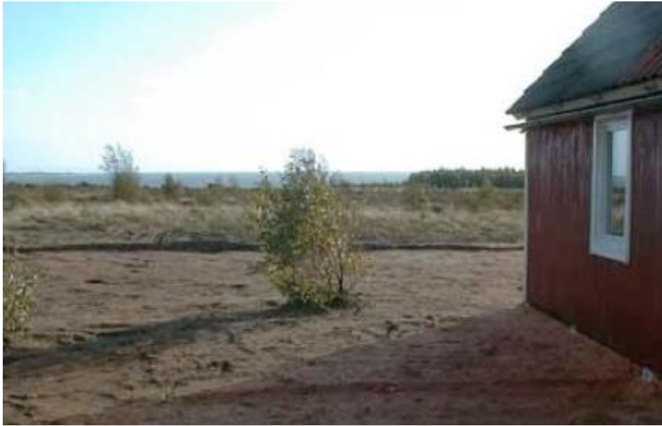
Figure 1. Surfaces around the house during the DEMOEX-exercise have been removed.
