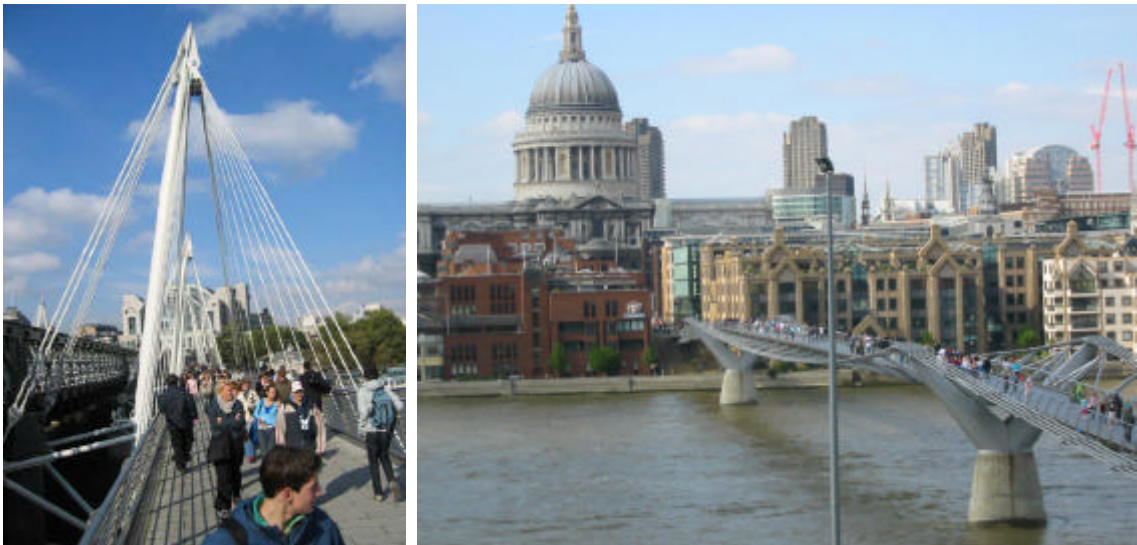
Figures 253-254. The New Pedestrian Bridges Give the Route Its Identity and Superb Views of London
