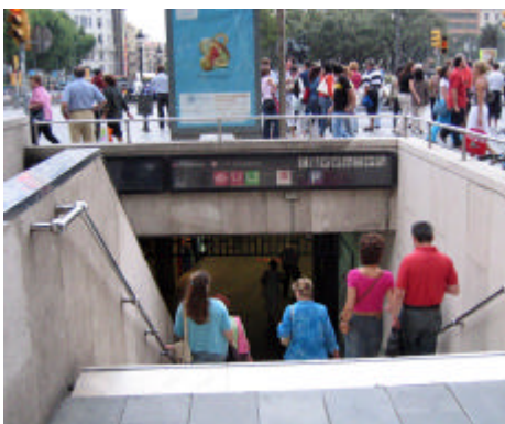
Figures 311-312. Rivadeneyra Metro Entrances (Missing the Usual Identification Pylons) Plaça Catalunya
