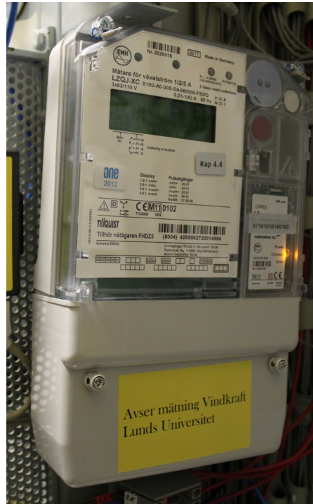
Figure 5.5: Electricity meter of type EMH LZQJ-XC which is mainly used in the field test.
