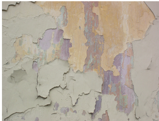
Figure 2. This detail of a plastered facade, from a farmers house in the coastal region of southern Sweden, shows many of the old layers of paint in many different colors.
