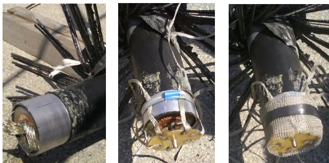
Figure 2: Shielded connection to the extruded HVDC power cable. The armour of the power cable has been opened and the standard coaxial cable is connected to the inner conductor and the lead sheath of the power cable.
