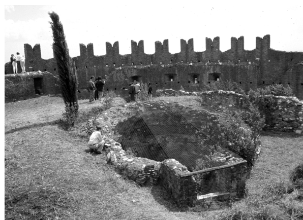
Fig. 35. The tomb of Caecilia Metella. The top of the drum with remains of a broken vault in the centre. Photo by N. Hillbom 1998.
