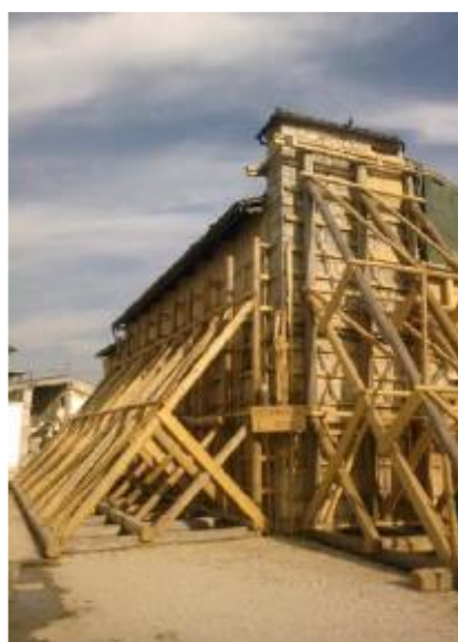
Fig. 5 - 6 Implementation of the protections in a restoration site in an area of high seismic risk (left). Shoring at a yard provisional reconstruction after the earthquake (right).
