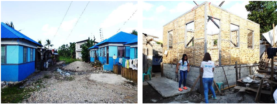
Figure 4.21 Agency-driven reconstruction on-site carried out by HFHP in Barangay Poblacion, Burauen. The housing typology and construction system of We Effect pilot housing were replicated. The owner decided to increase the height of the housing without receiving technical advice on housing adaptability for future expansion. Pictures: by the author, March 13/2015
