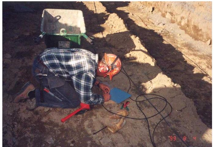
Figure 4. Installation of resistivity electrodes.
