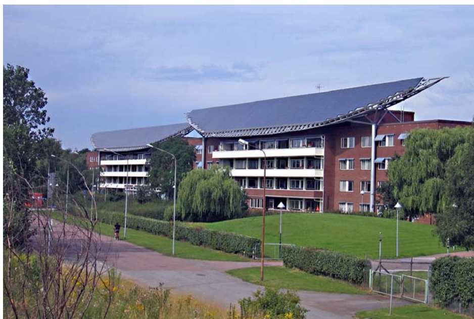
Figure 22. The solar cell installation at Sege Park (Solar Region Scania)
