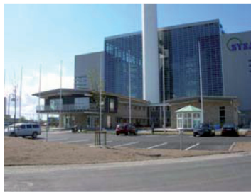
3231.2 New Maglarp Church today at Sysaw as a conference facility in front of the industrial plant.
