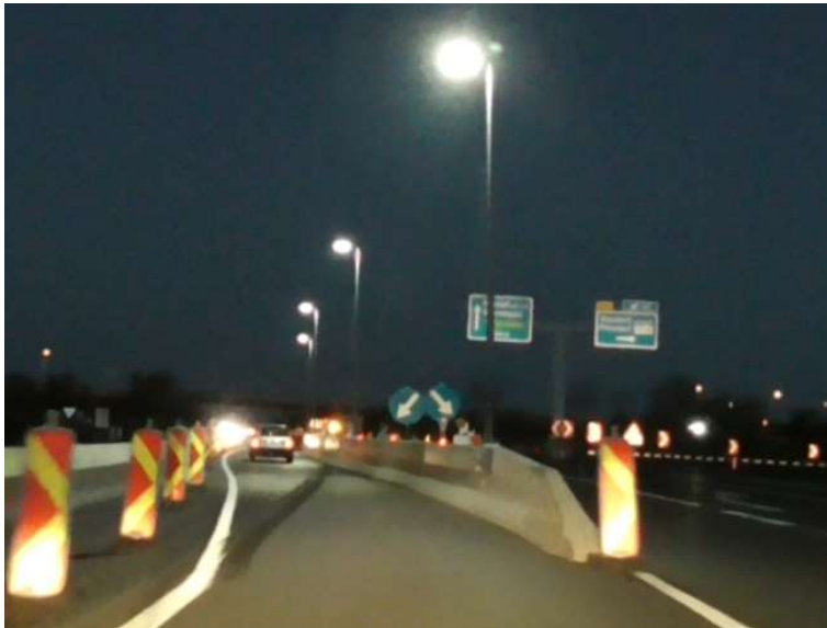
Figure 30: Illumination of critical zones
