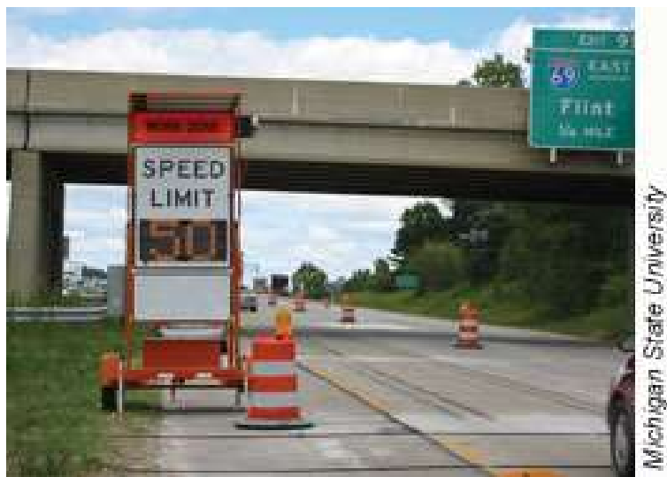
Figure 24: Variable speed limit sign in work zone
