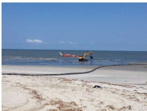
Figure 5. Beach nourishment action implemented as part of the the recent coastal protection works at Costa do Sol beach in Maputo City. From and by permission of Fátima Ismael.
