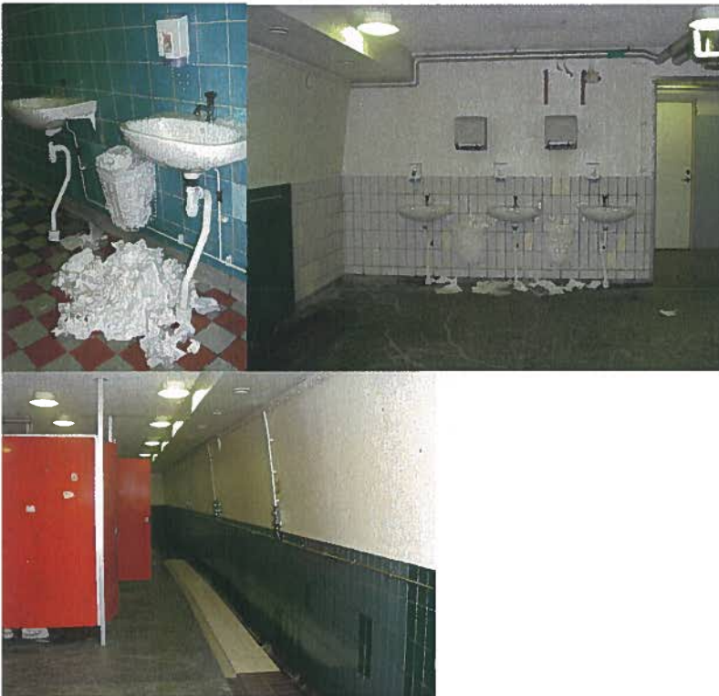
Figure 12. Washroom in Malmö Stadion.
