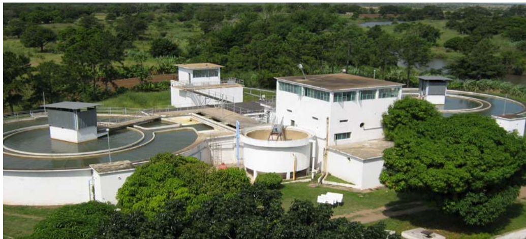
Figure 1: One of two treatment plants at Aguas de Moçambique. © AdM
