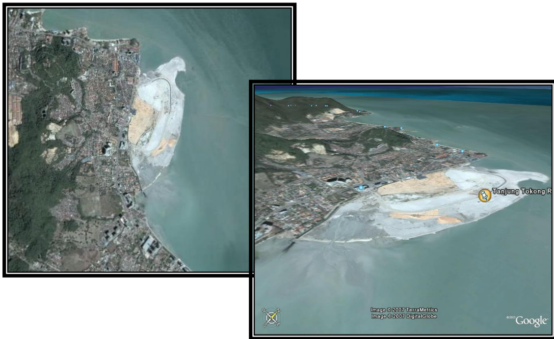
Figure 4 : View of the Tanjung Tokong Land Reclamation Project (from Google Earth)
