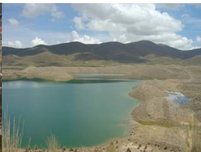
Figure 15. Dam formed through dredging by ESTALSA, pH 3.07
