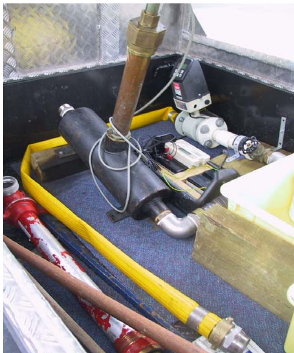
Figure 23 - Equipment placed in the trailer (Kjellberg 2006)
