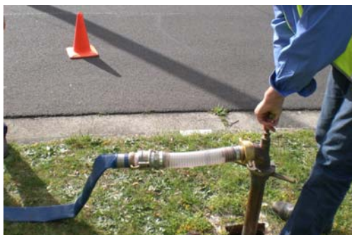
Figure 22 - Placement of standpipe in hydrant (Kjellberg 2006)
