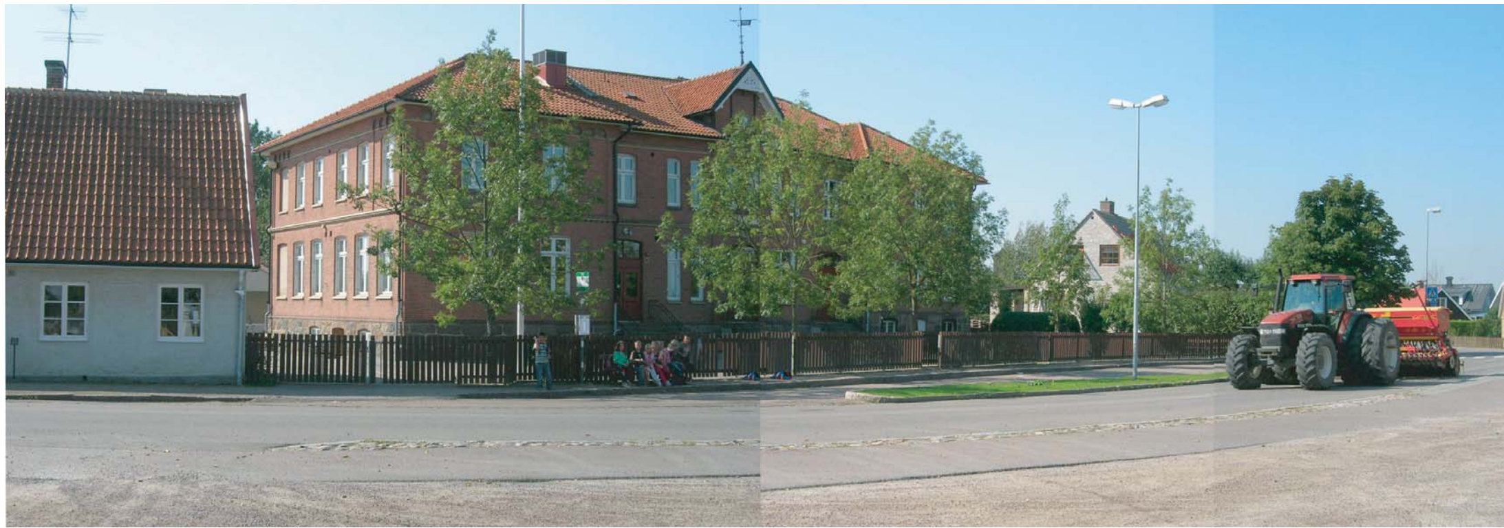
The school in Kattarp.
