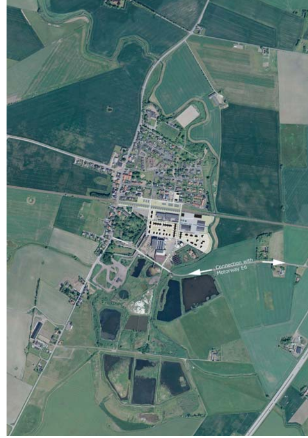
Phase 1 - the factory area.
