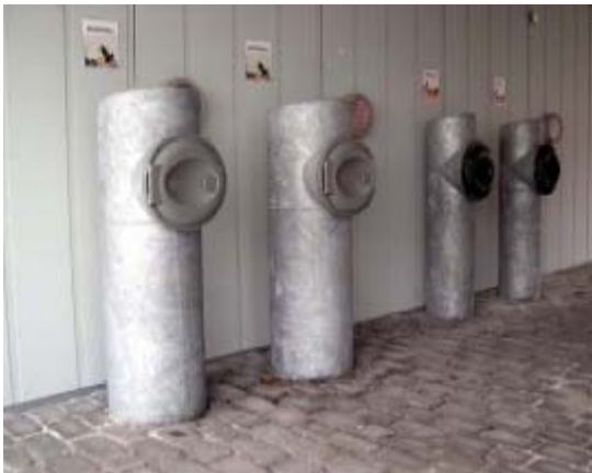
Figure 4-5 Vacuum Waste Collectors (City of Malmö, 2006)
