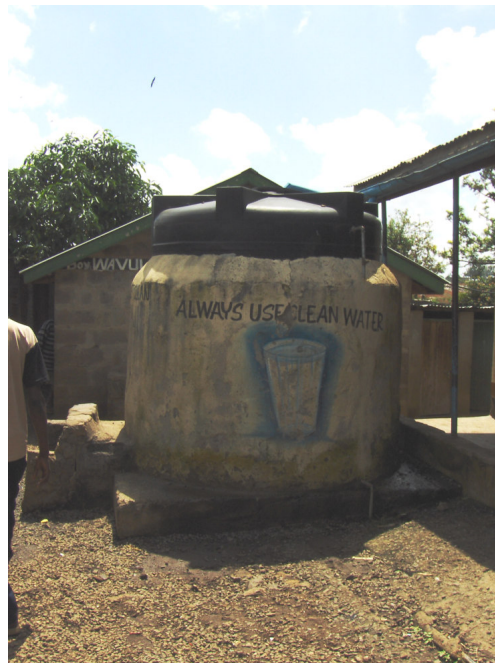
Educational water tank at school in the Korogocho slum
