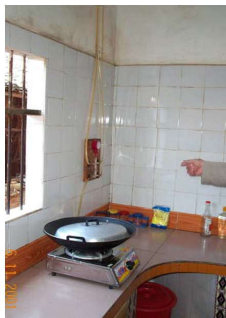
Figure 3-12 Biogas for modern cooking in Guangxi Province, China
