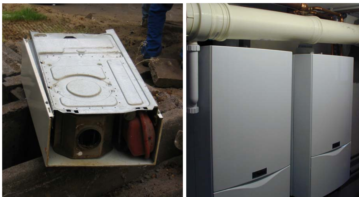
Figure 4a&b, Old boiler and new GCH boiler
