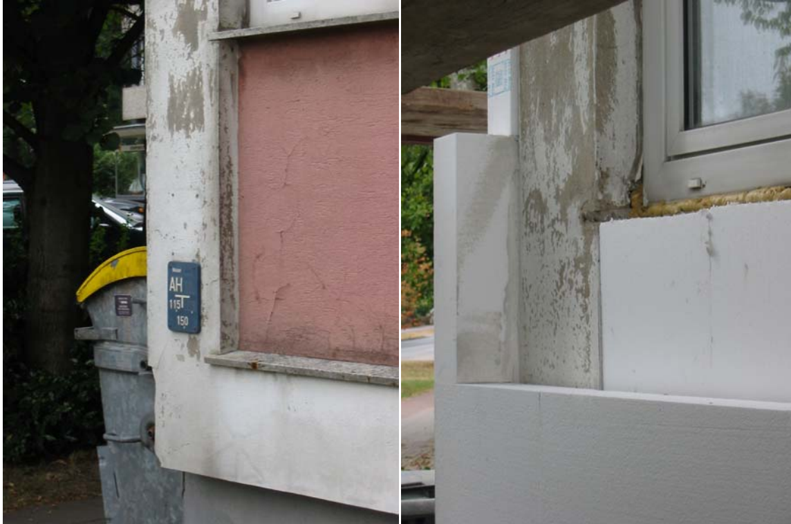
Figure 2a&b, Corner of the house without and with insulation layer
