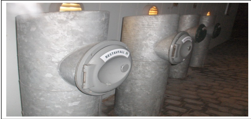
Figure 3-3: This waste sorting facility in Västra Hamnen , Malmö is located in a lighted, public and viewable location to motivate commitment to proper sorting.
