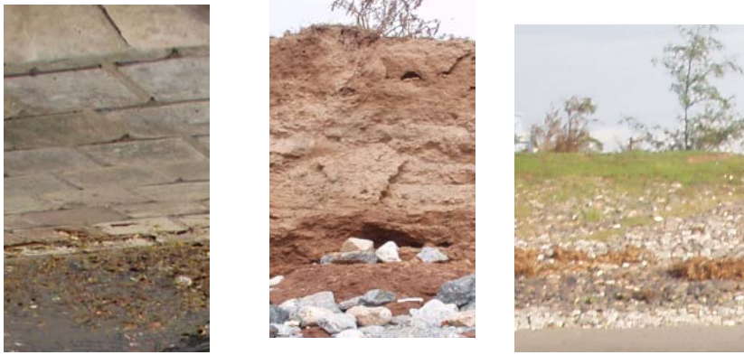
Figure 8 Dyke structure at station P1, P2, and P3.
