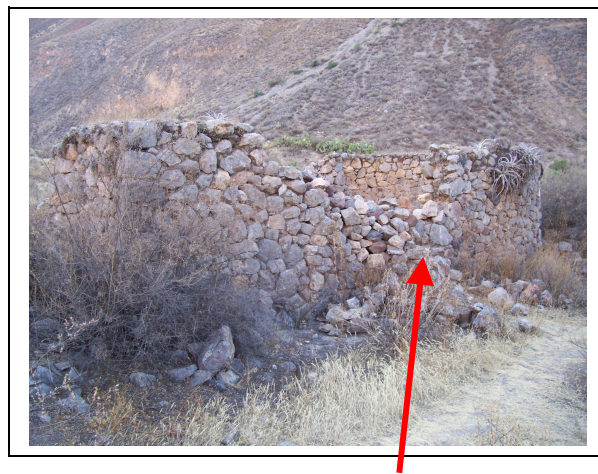
Previous entrance to the enclosure?
